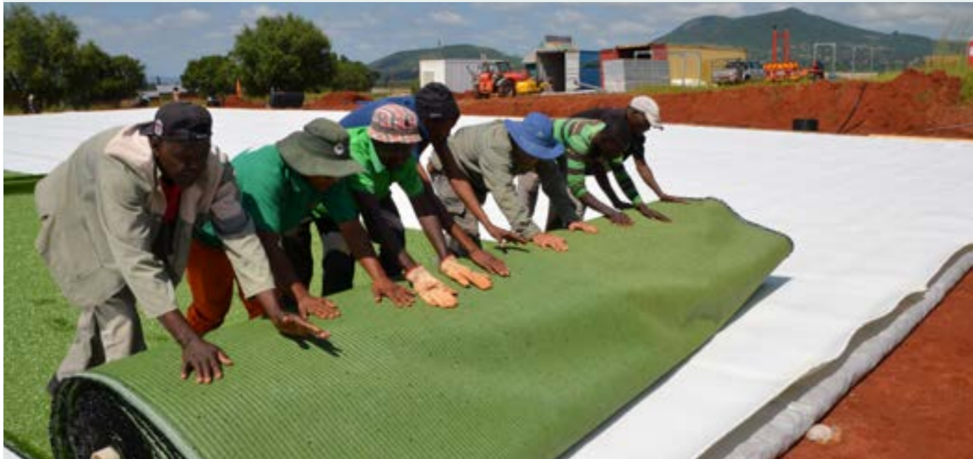
FDW12SA01 - A GREEN SUSTAINABLE AND SAFE WATER SOURCE - SOUTH AFRICA
