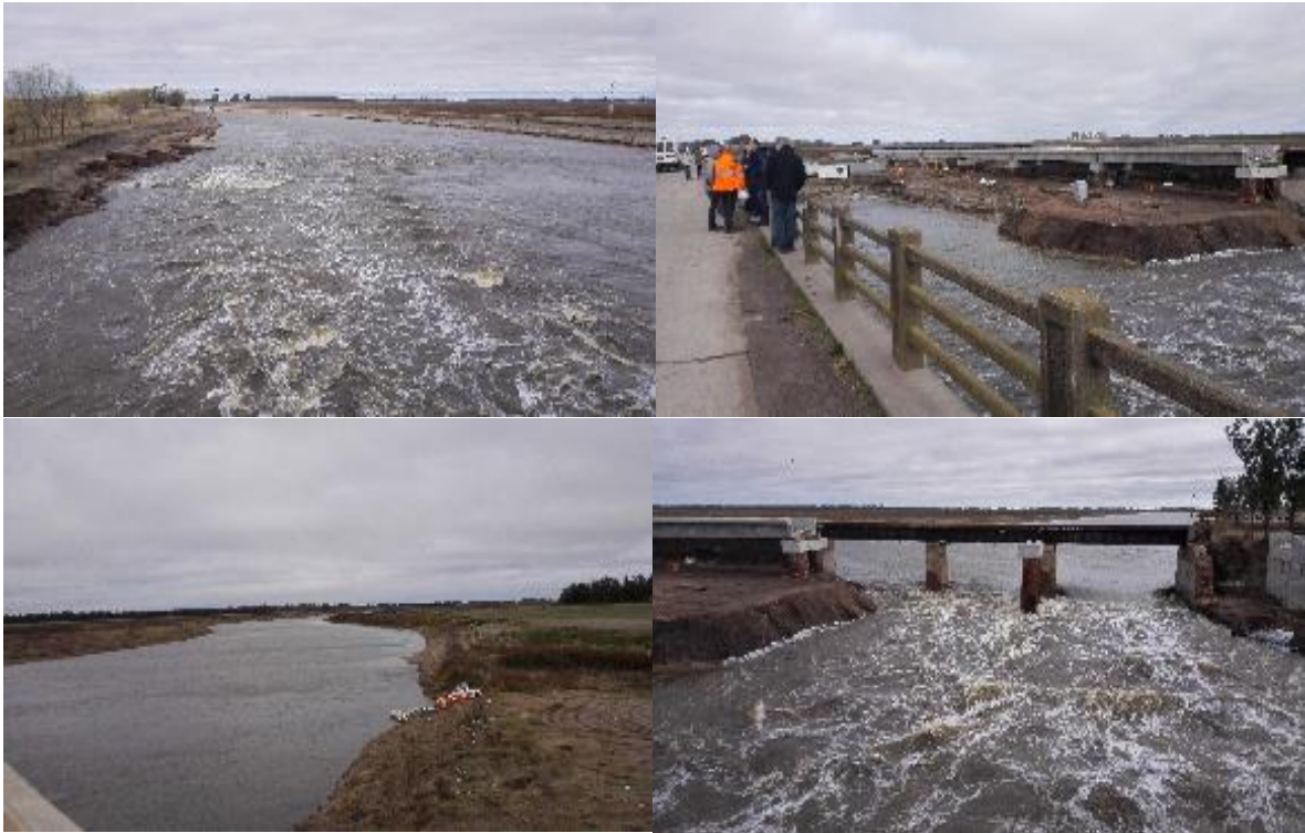
Figure 3-12 work in progress
