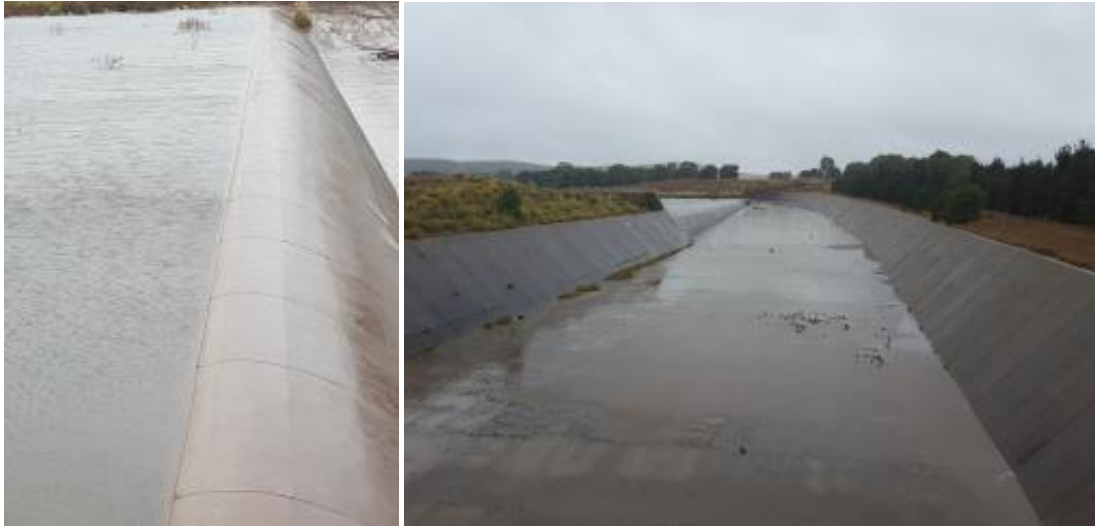
Figure 2-7. Spillway and Channel downstream 31 May 2016
