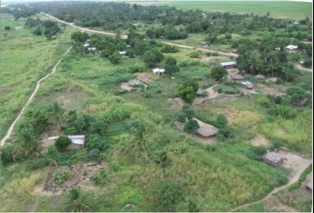
The dikes visible in this picture do not show major flood damage and seem to be over grown with grasses for several years.
