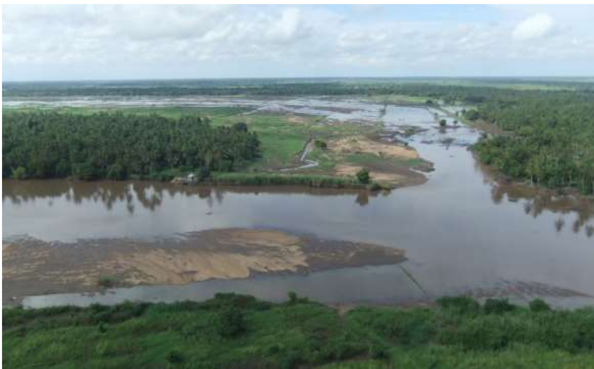
Figure 17 – Intabo Intake Station, Canal and Breach
