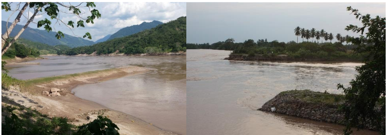
Picture 3-3 Groynes as an effective solution against erosion (Shapaja) and in San Hilarion inflow of Sisa as wrong example
