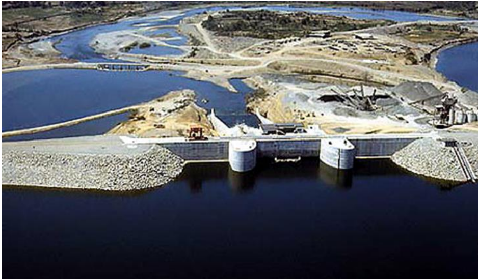
Picture 1-4 Poechos Dam (source:water-technology.net Image courtesy of Energoprojekt)
