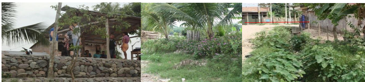
Picture 3-6 Protective measures in Puerto Ambares/ Juanjui with in red line the inundation line
