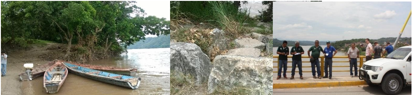
Picture 3-9 Bella Vista without and with flood protection and bottle neck in the river at the suspended bridge location
