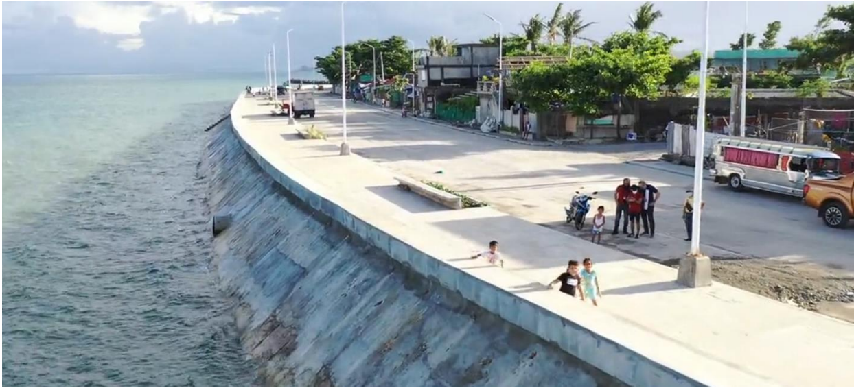
Figure 2-4: Seawall in Virac
