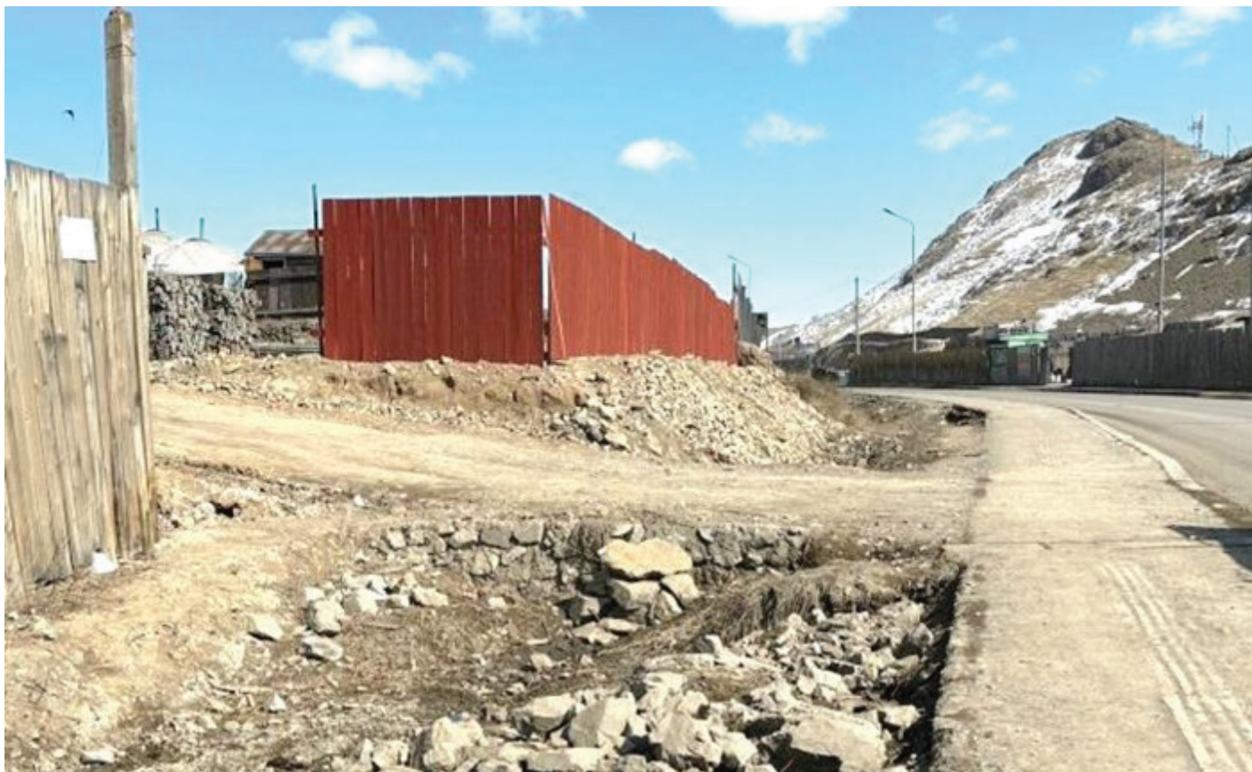
Figure 14b: Flood drainage facilities (culvert and channel) in "Gants Khudgiin Am" watershed (Source: photo by Chinzorig, IGG, MAS)
