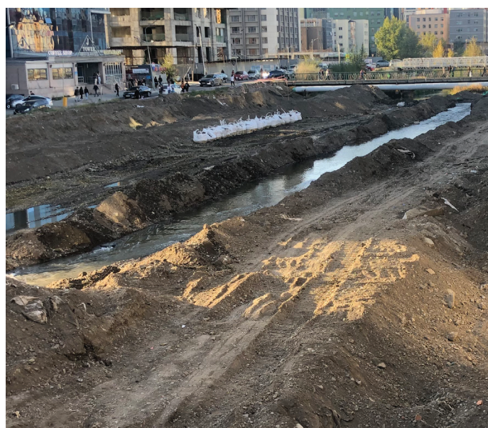
Construction activities in the Selbe River ongoing Revival plan
