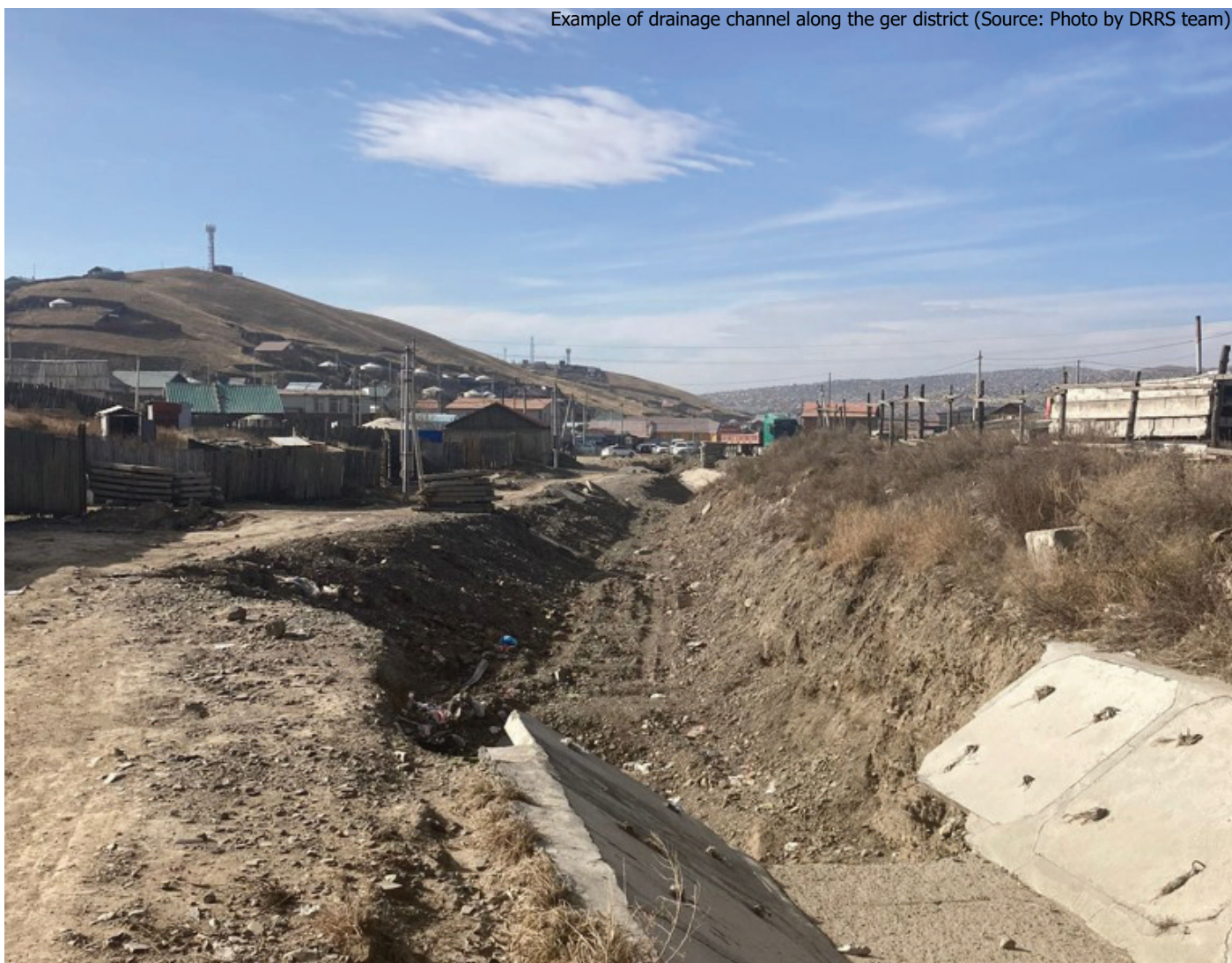
Figure 14b: Flood drainage facilities (culvert and channel) in "Gants Khudgiin Am" watershed (Source: photo by Chinzorig, IGG, MAS)
