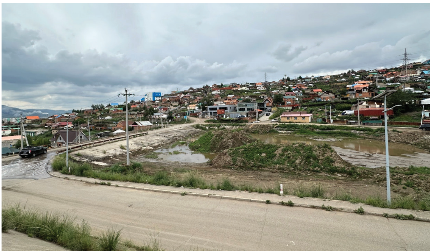
Figure 27: Sambalkhudev retention basin full of sediment (Source: Photo by Chinзориг Сухбаатар)
