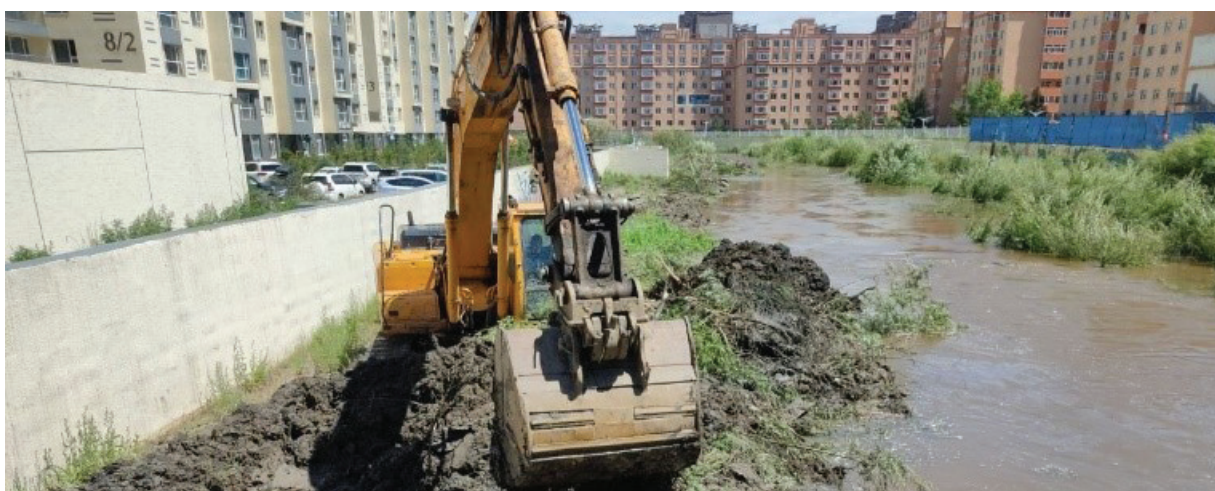
Figure 28: Excavation work in the Selbe River on June 23, 2024
