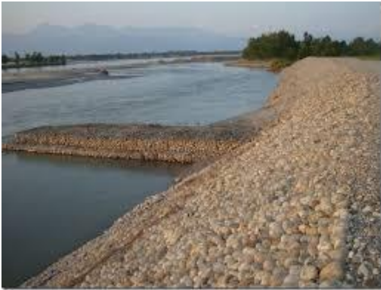
Photo: example of a levee and river training works.
