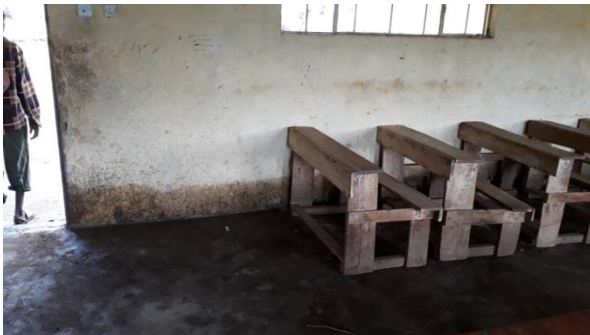
Flood mark in School in Ngambo irrigation scheme near Marigat Photos of the study area.
