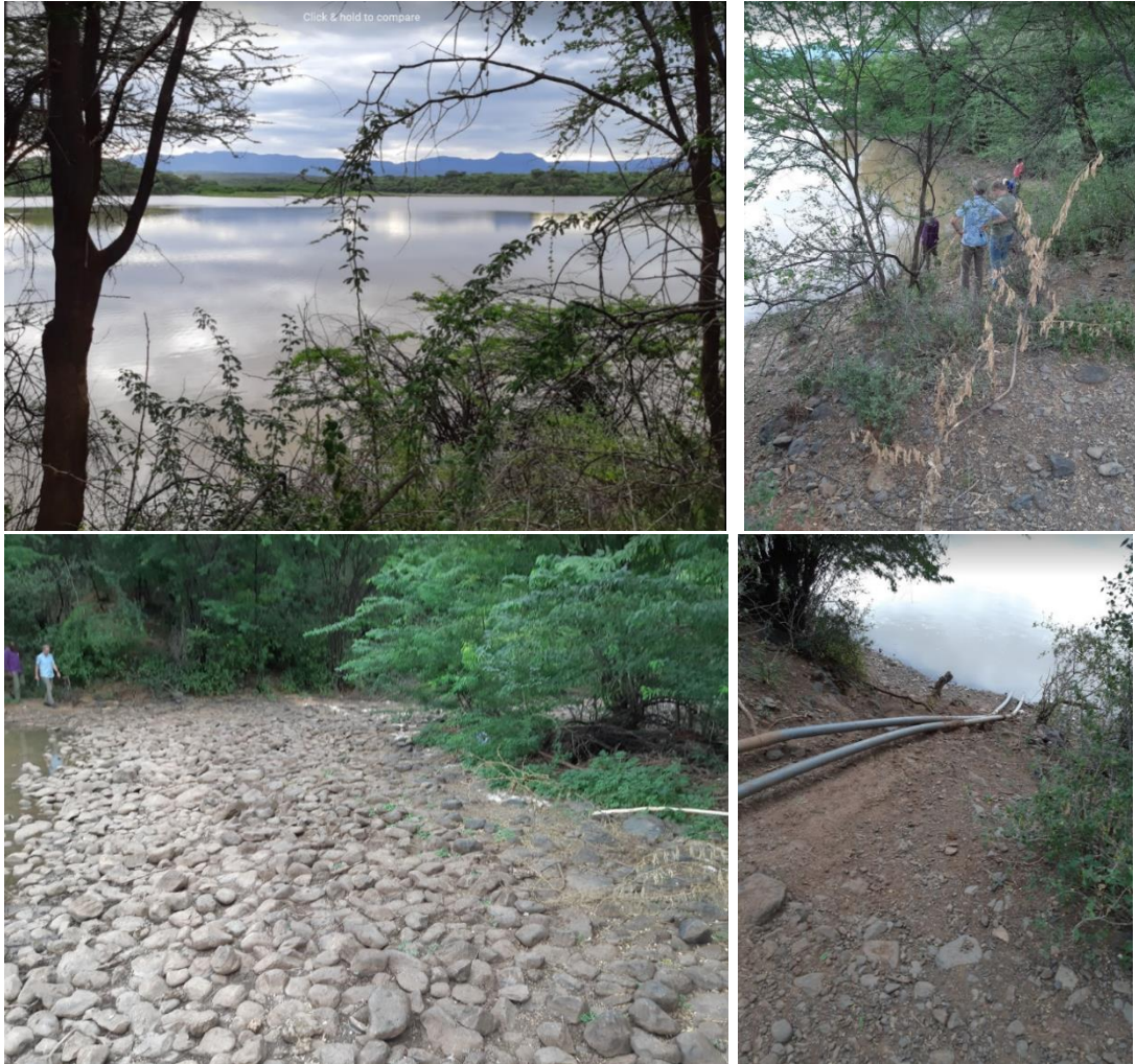
Photos: Chemeron Dam (reservoir, bush on embankment, spillway, water abstraction)
