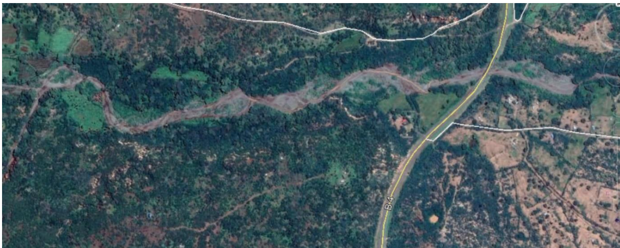
Figure 10. Area directly downstream Chemeron Dam. The valley at risk is some 30m deep, 2.2 km long from dam to road, and has small scattered settlements.
