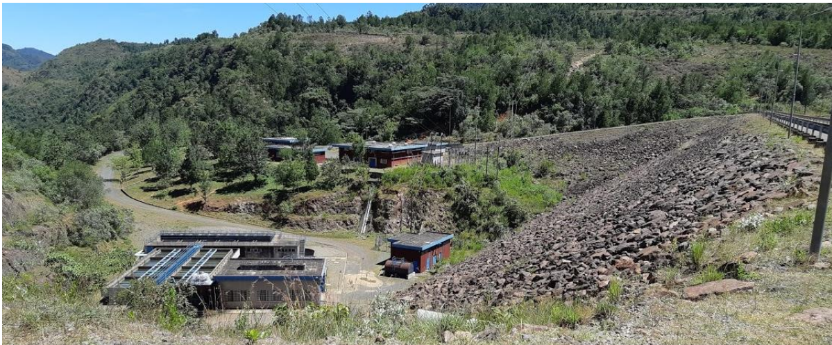
Photos: Kirandich Dam, Phase I (Embankment, reservoir, water treatment plant).
