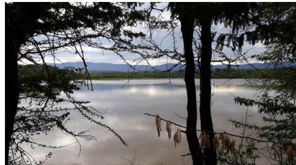
Trees overgrowing the Chemeron Yatoi Dam
