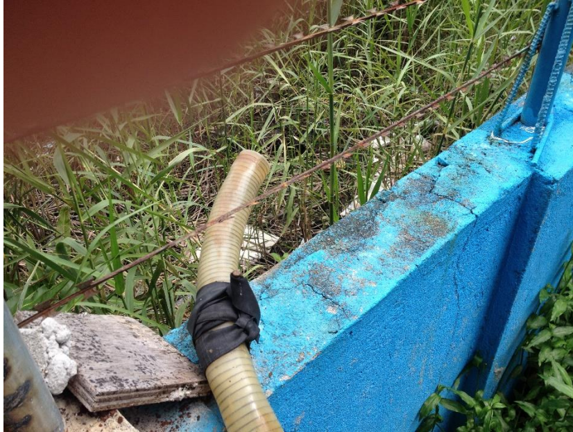
Figure 4.6: RO reject draining to the nearby field (not in use during the visit)
