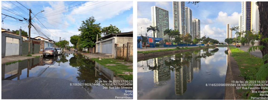
Figure 4: Street floods at high tide
