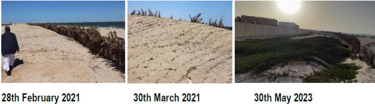
Figure 10 – Development of biological fixation of dunes in Nouadhibou (Dune restoration project in Mauritania). These images are included in the guide biological fixation of coastal dunes by halophilic plants 16 .
