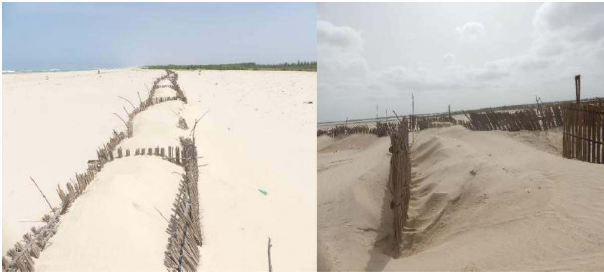
Figure 7 – In a number of iterations the design of the wind breakers used for dune restoration in Senegal have been improved. Orientation and permeability of the wind breakers is important 13 .
